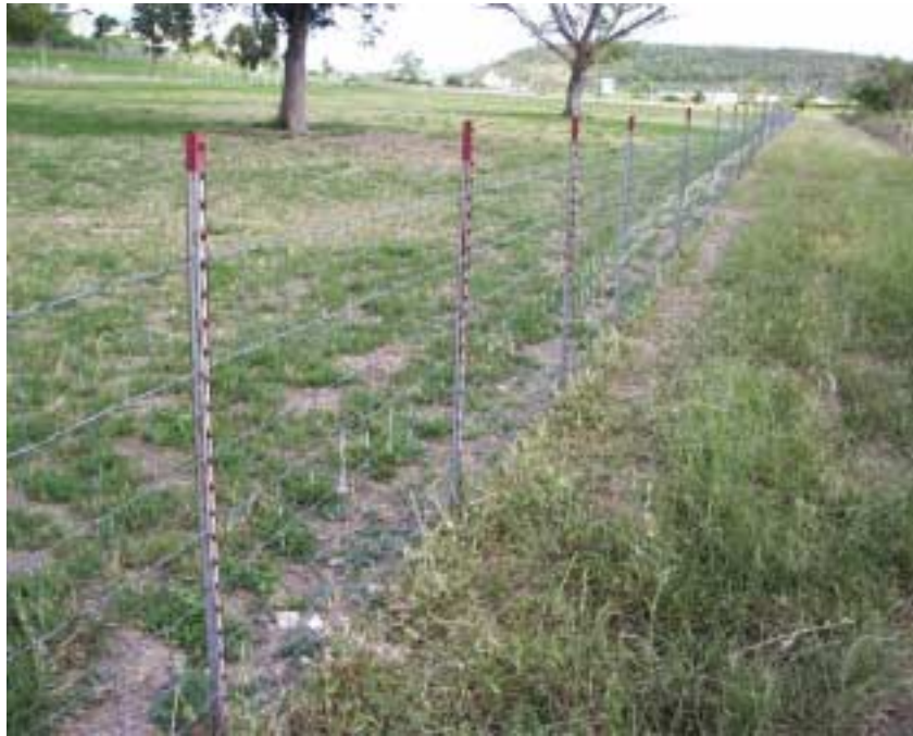
Figure 1. Wire fence supported by metal posts. Fence is attached to the posts by metal clips after the posts are pounded into the ground.
